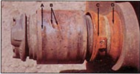
Fig. 12: Adapter has been displaced to inboard end of bearing. Adapter thrust shoulders have been in contact with outer race over the load zone outboard (A & B) and with the backing ring and journal fillet radius inboard (C & D) indicating multiple displacements.
